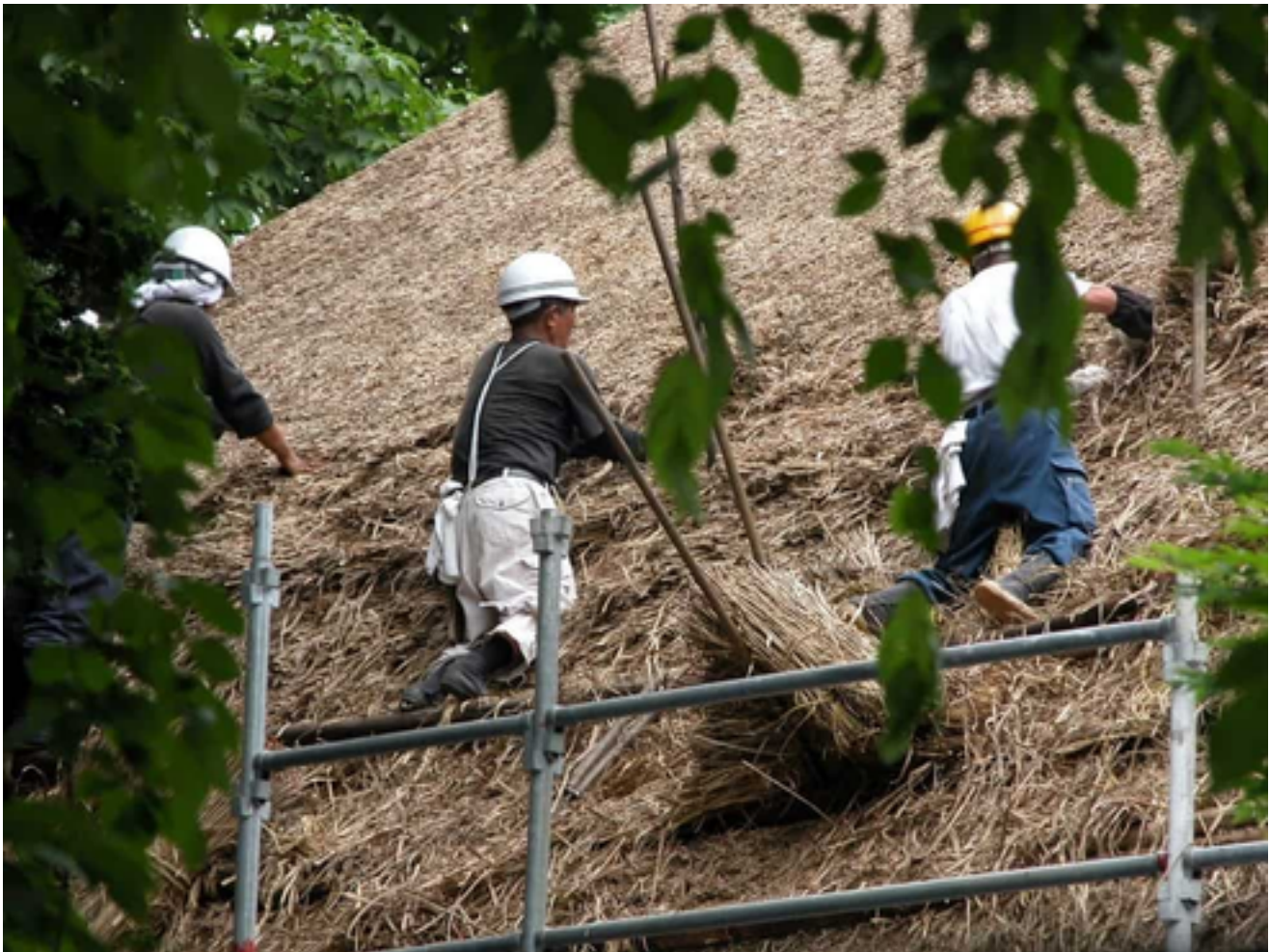
Replacing the thatch roof at Ishiguro Samurai House
